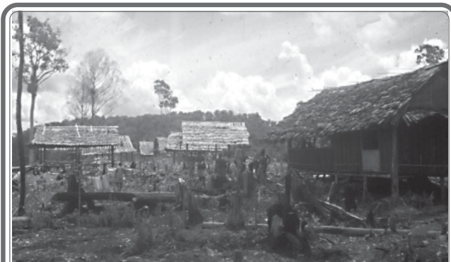
The house where the devil appeared to Salapan
