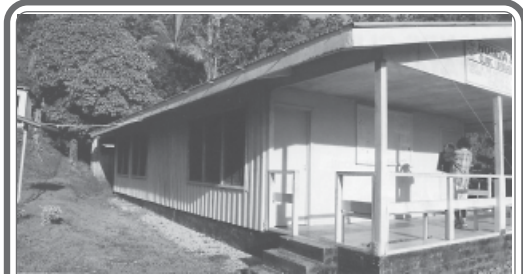
The permanent clinic building at Honoa completed in 2005 with the help of AusAid
