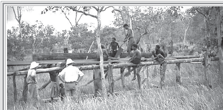
Pitsawing the timber
