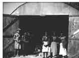
18 A Quonset hut for the press
