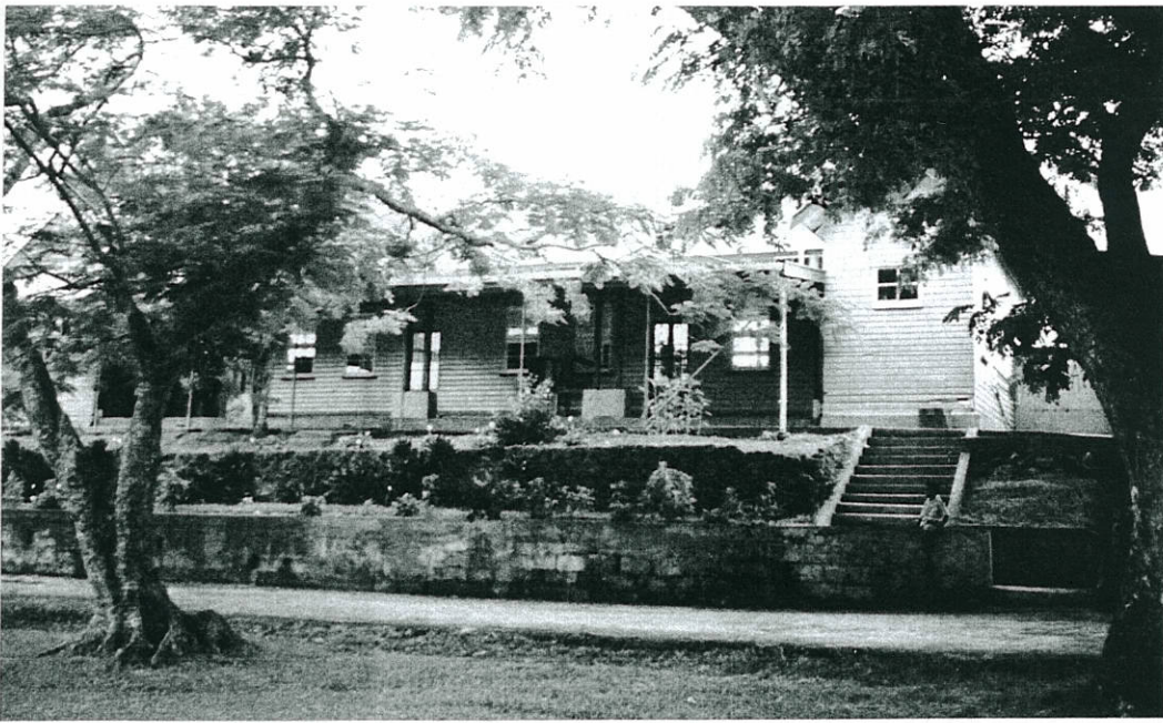
The former Indian School at Samabula as it was in 1995—still used as a school
